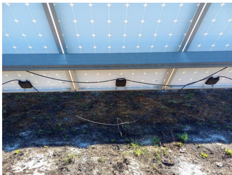
Figure 26. Overheated DC connector
