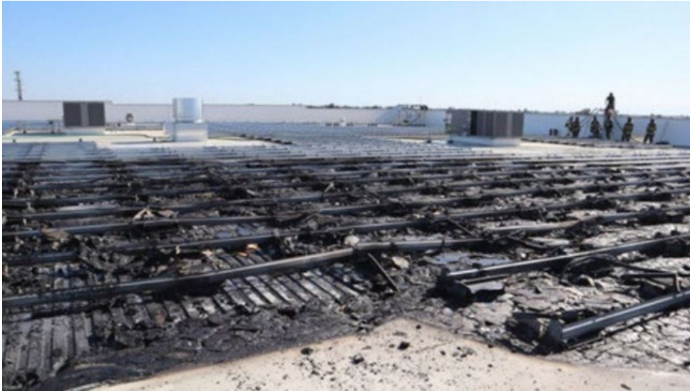
Figure 13. Solar farm after fire. Source: https://kmph.com/
